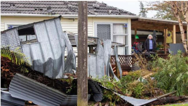
A woman surveys damage to her Levin property including parts of a shed blown across the street during the May tornado. Photo/ NZ Herald
